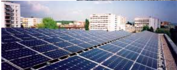
Photo: AS Engineering AG, Bern
